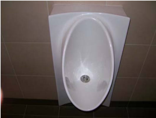
Figure 17: 0 litre/ flush 'K ohler sensor' urinals found in the Fipke Centre.
